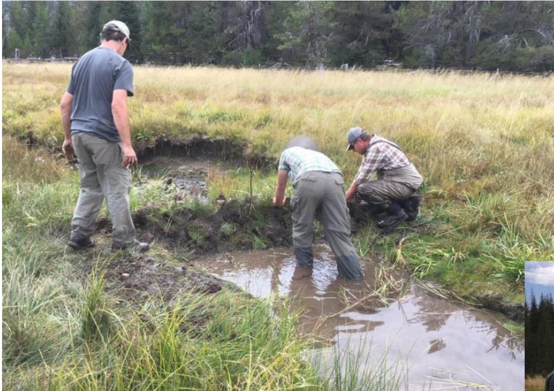
BDA maintenance - repacked dams from meadow materials
